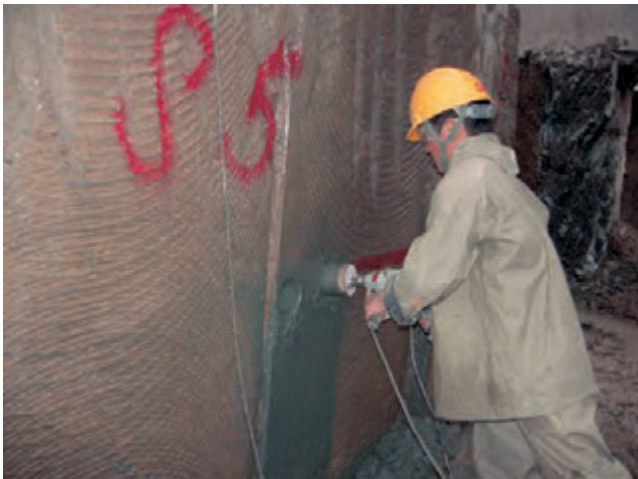
Horizontal core sampling with a hand-held drill
