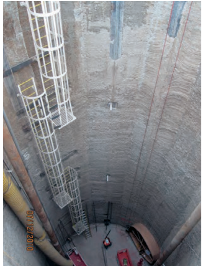
CSM-wall for start shaft microtunneling (USA)
