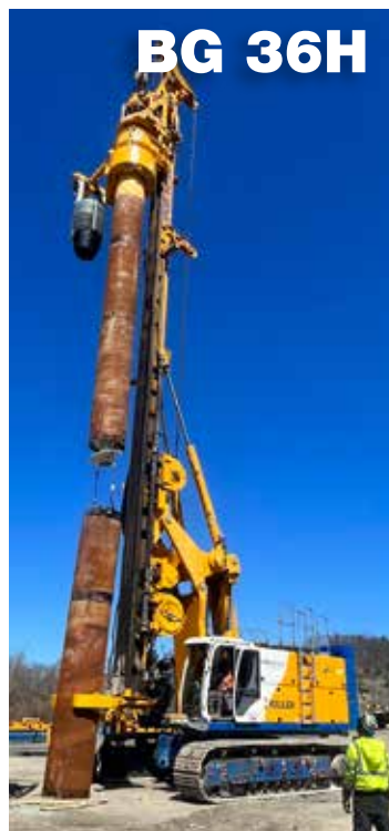
CCFA Cased Continuous Flight Auger
