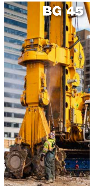
CSM Cutter Soil Mixing
