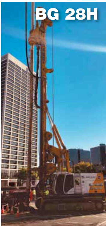
FDP Full Displacement Pile
