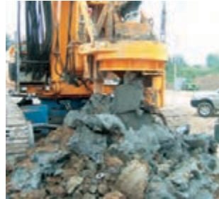
Continuous conveyance of spoil with CFA (as a comparison)
