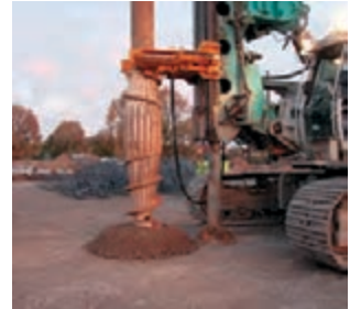
Negligible conveyance of spoil with FDP
