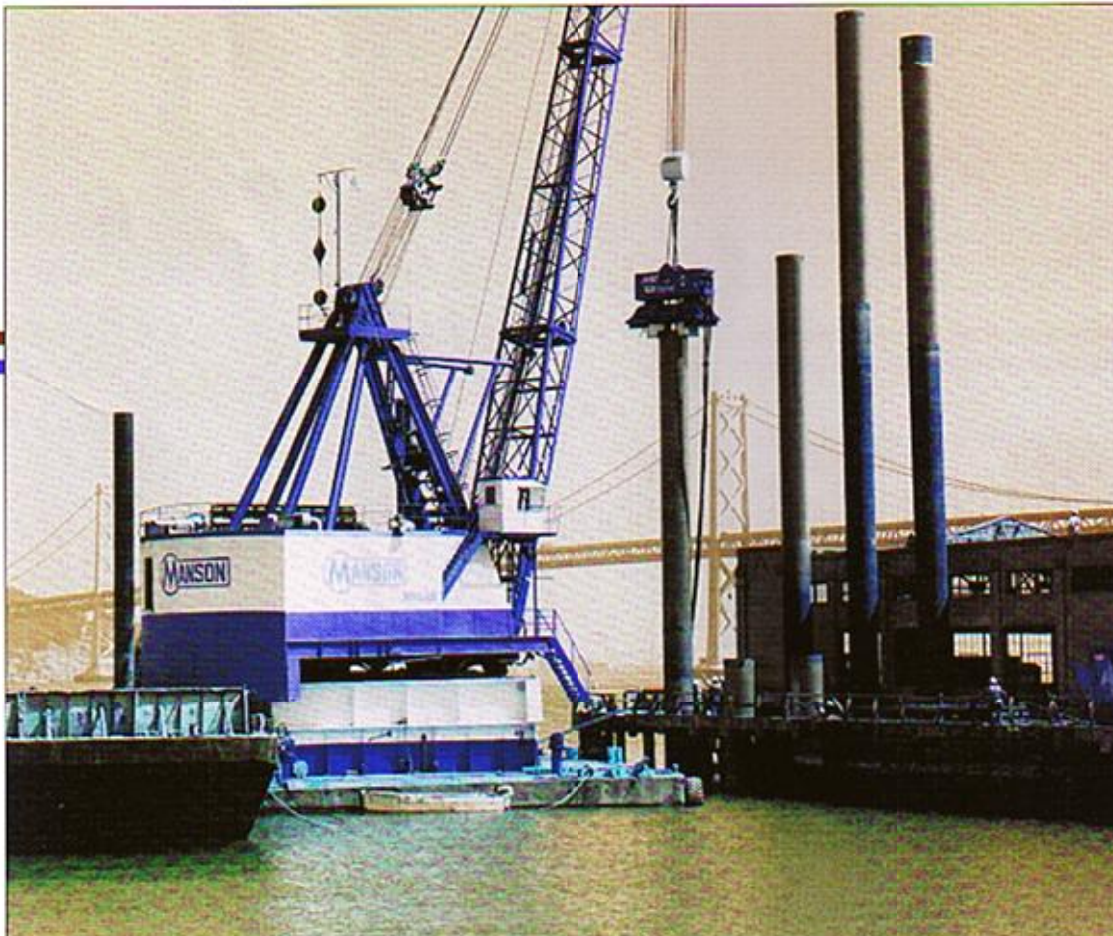
Model 1600 driving 150' pipe on San Francisco wharf project
