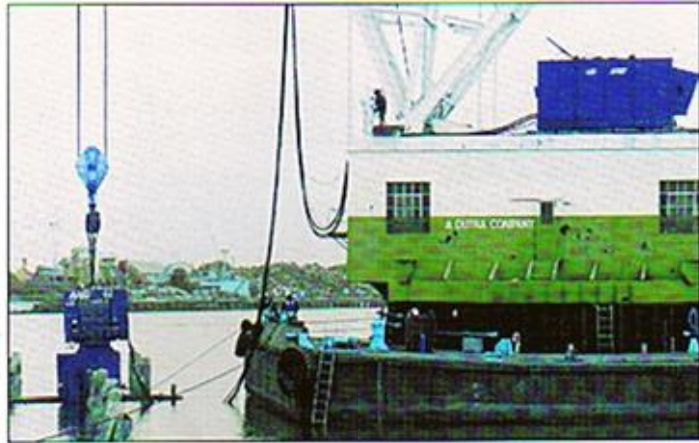
Model 450 Extracting 24" Concrete Pile
